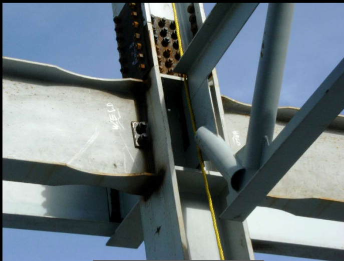
Prequalified Moment Connection: Reduced Beam Section
