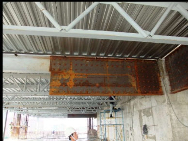
Connection of Steel Truss to Column
