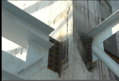
Connection of Steel Truss to Column
