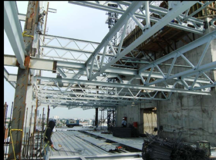
Connection of Steel Truss to Column
