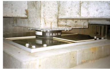
Sliding bearing for elevator weight
