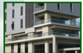
Civil Engineering Research Building of NTU
