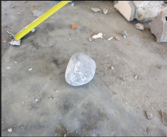
Improper size and type of aggregate
